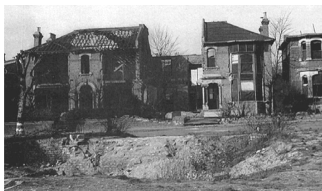
Breakspears Road: damaged houses, front exterior Council flats replaced bombed houses
