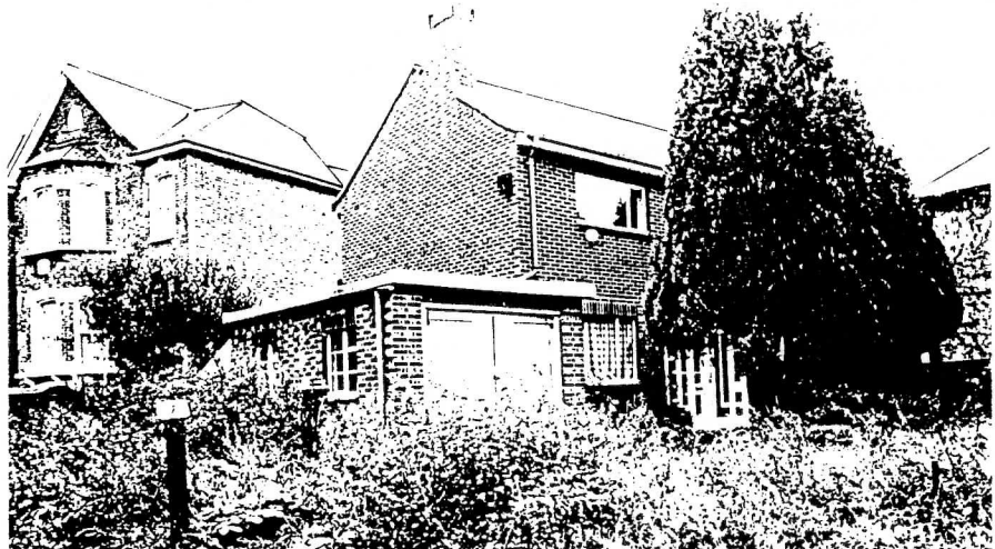
199 Wickham Rd.-Application for demolition is under consideration.
