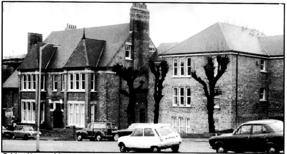
Bridge House, Montague Avenue
