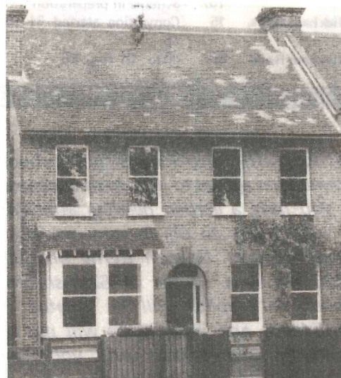
Hilly Fields Crescent Refurbished by the Council.
