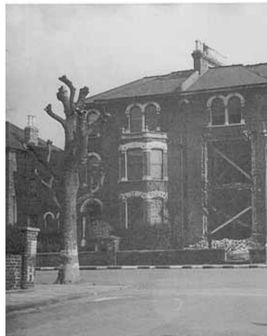
Damage to 103 Breakspears Road. 13/3/1944
