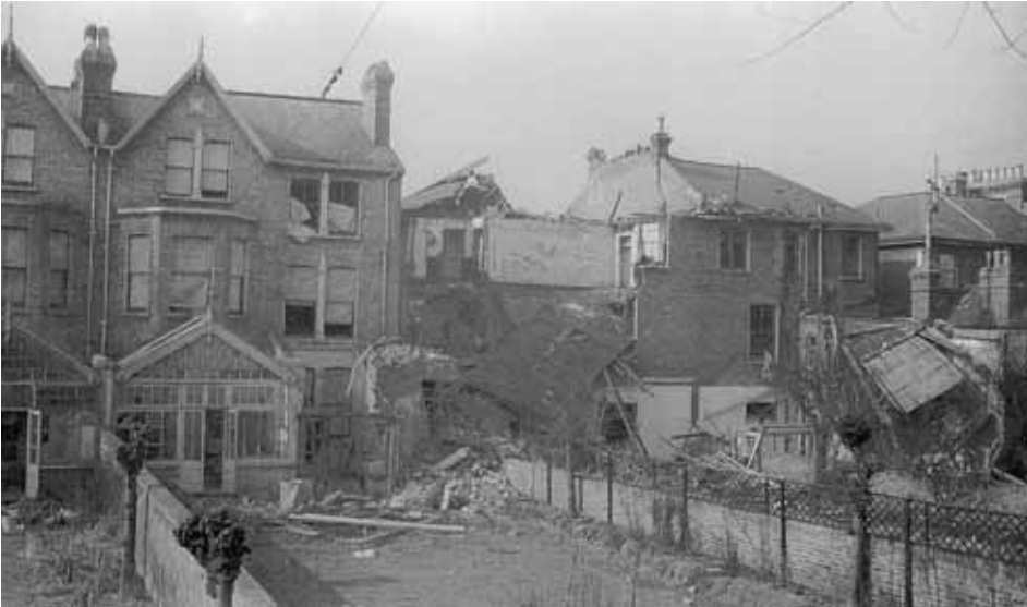
Bomb damage to 67 and 69 Breakspears Road (bombed in November 1940). 5/4/1941
