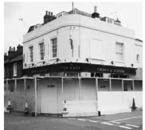
. . . and after stripping the tiles
