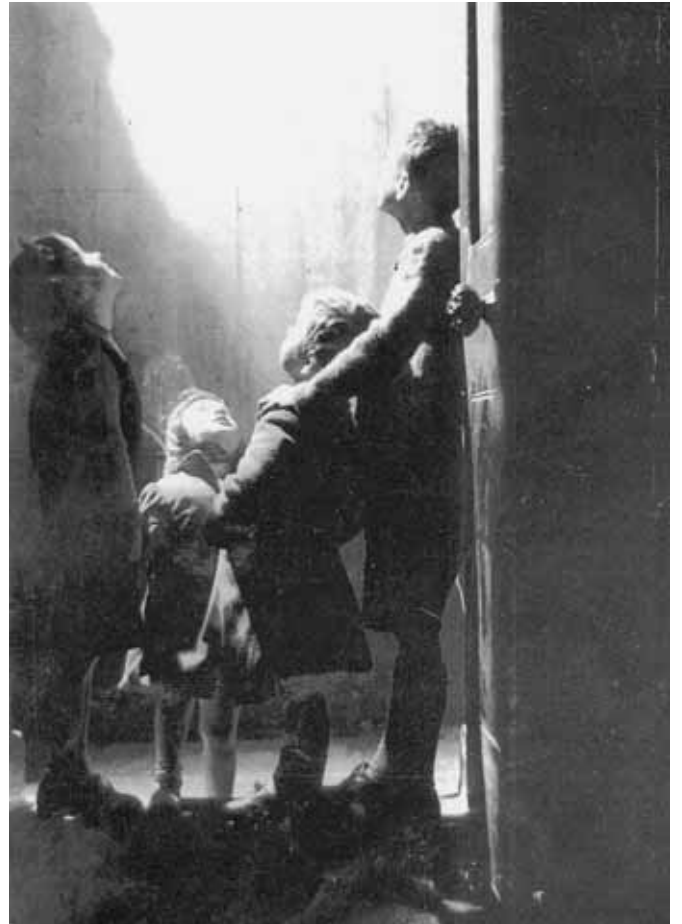
Testing street lighting, Malpas Road. 6/1/1944
